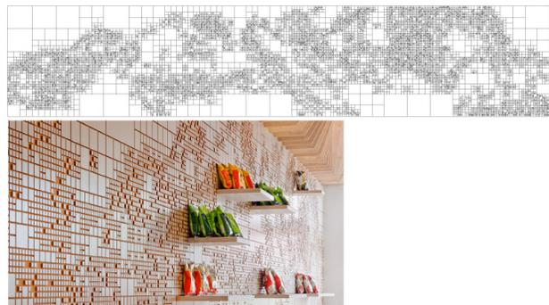
Figure 4. Freeland Buck's CNC-milled wall surface at Earl's Gourmet
