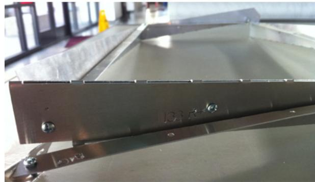
Figure 3. The frame was made of two interlocking, folded aluminum pieces.
