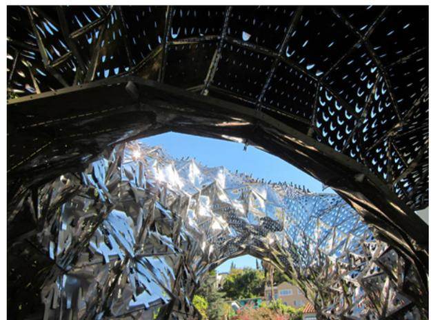
Figure 10. The project was made of over 14,000 bimetal pieces.
