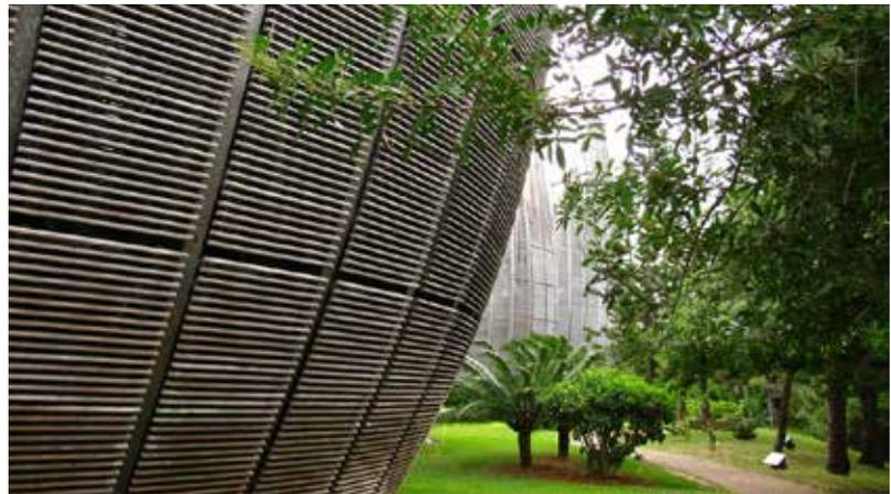
Figure 5: The *iroko* has begun to grey, helping to ground the structure to its surroundings (Flickr user MomLes).
