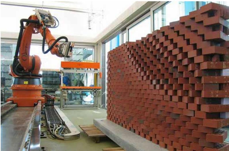
Figure 3: Programmed Wall, 5-axis robot building one of the wall scripts.
