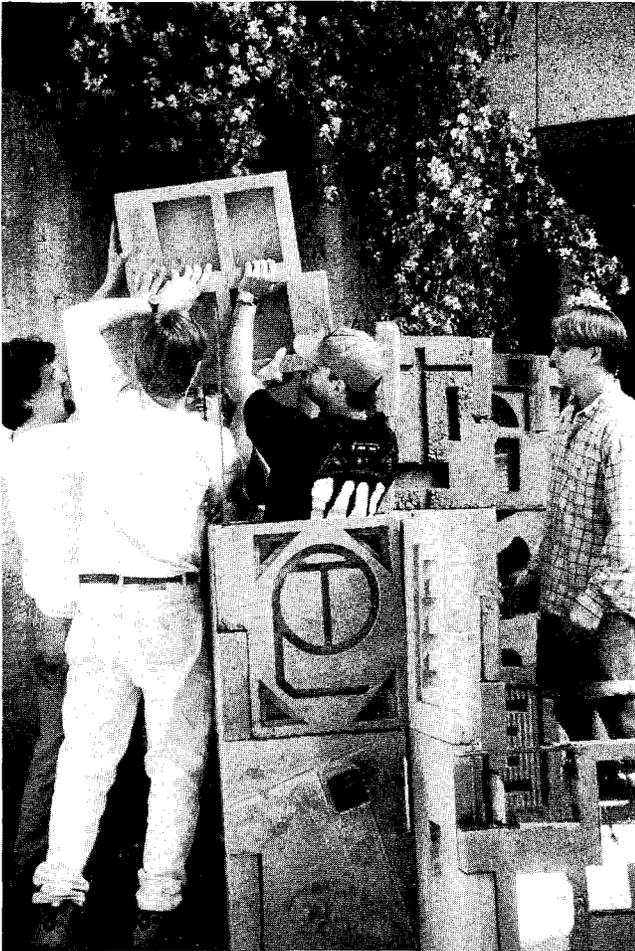
Fig. 2. Students assembling precast concrete wall
