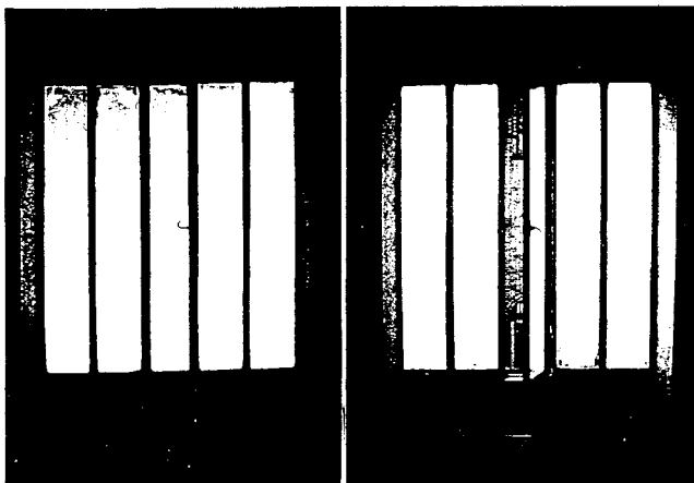
Fig. 1. Le Corbusier, Villa La Roche, Paris, 1923: Vitrage d'usine (factory glazing), with operating panel closed (left) and open (right). (Photos: H. Sobin).
