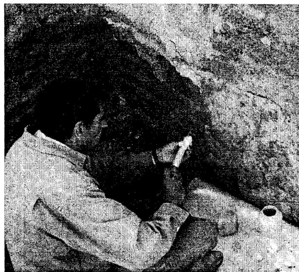
Fig. 6. Stabilization and consolidation of plastered wall surfaces. Frank Matero. Photo Lindsay Falck .
