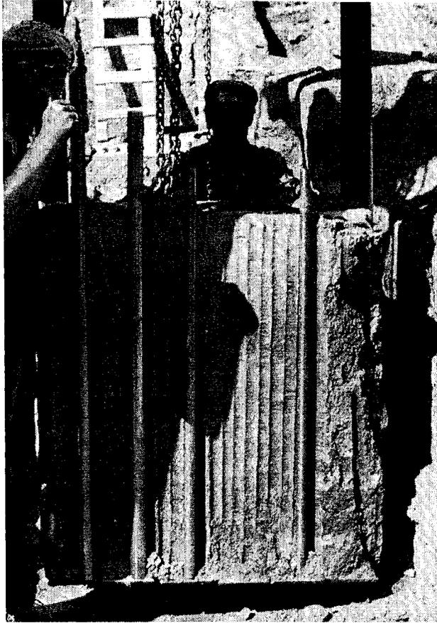
Fig. 8. Detached wall panel with cam-lock tubes. Photo Lindsay Falck.
