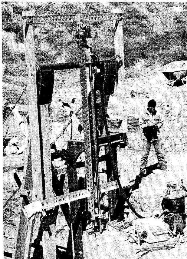
Fig. 7. Rig complete with drill frame and vacuum. Photo Lindsay Falck.
