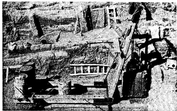
Fig. 1. Lifting rig with detached wall panel suspended in steel lifting harness. September 23, 1996. Photo Lindsay Falck.
