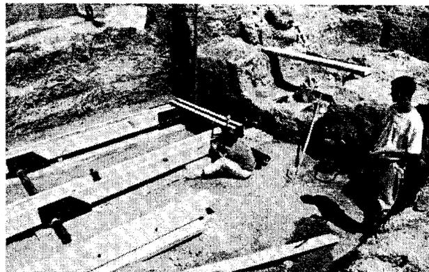
Fig. 5. On-site erection of Lifting rig ground beams. Caitlin Moore and Evan Kopelson. Photo Lindsay Falck.
