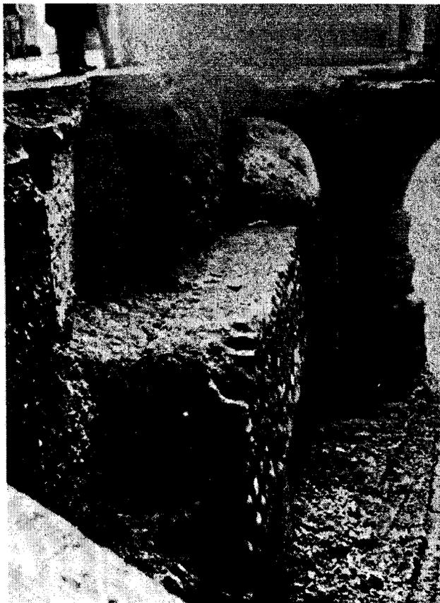
Fig. 16. Excavation of the Scaligeri moat under the fifth room of the gallery. The arches carrying the wall of the Napoleonic barracks were constructed in the nineteenth century. Scarpa introduced the foundations.
