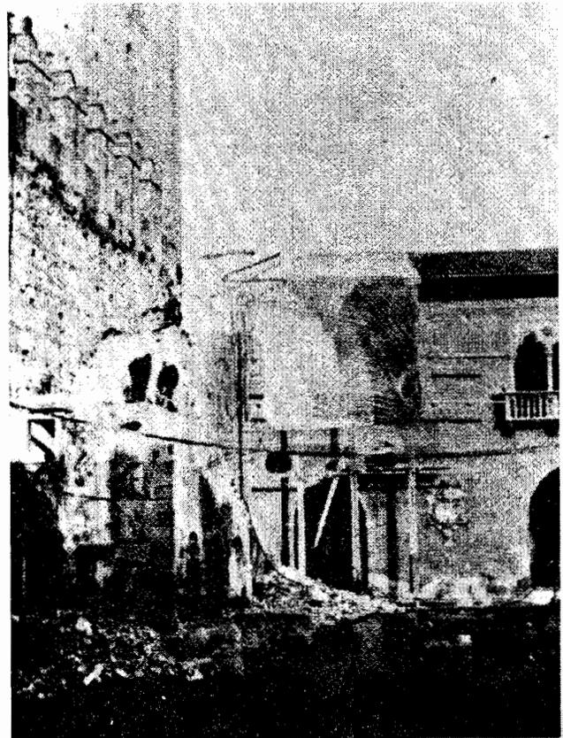
Fig. 15. Scarpa's demolition of the final bay of the Napoleonic barrack and the excavation of the Roman moat.
