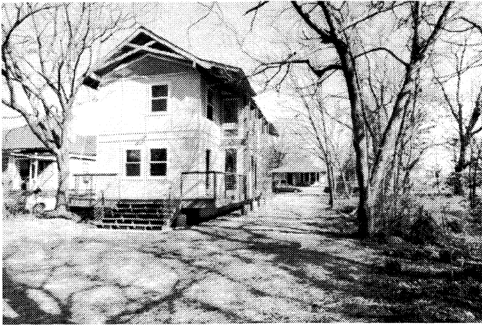
Fig. 6 Exterior photo showing the rear elevation of the house in context.
