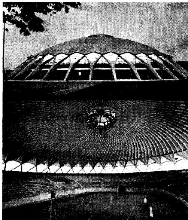
Fig. 6. Palazetto dello Sport, Pier Luigi Nervi, 1958. Exterior showing y-buttresses, and interior showing pattern of lamella dome.
