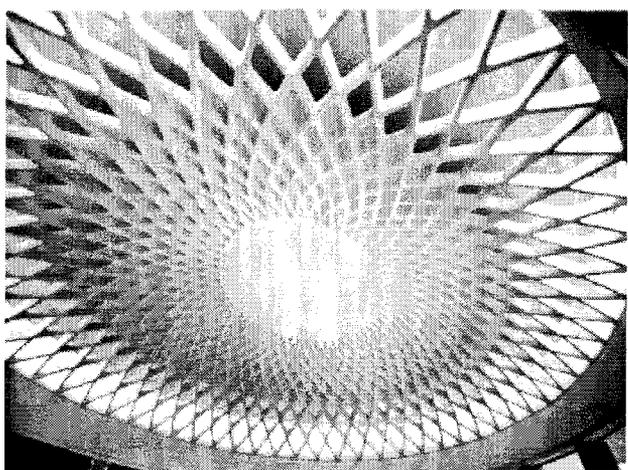
Fig. 5. Terme di Chianciano, Pier Luigi Nervi, 1952. Roof structure showing pattern of ferro-cemento formwork.
