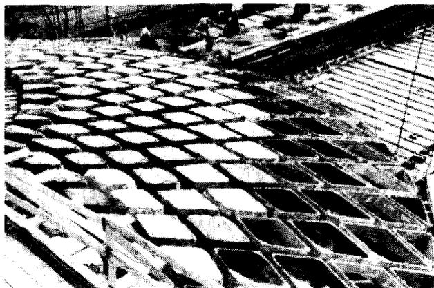
Fig. 4. Constructional system used on the lamella dome projects. Pans of ferro-cemento form a permanent formwork for the poured concrete dome.
