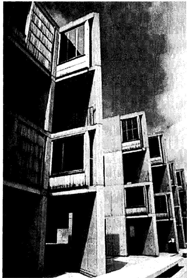
Fig. 6. 'Portico of Studies' from the courtyard. Concrete formwork joints show both division of floor slabs and an overall 4' x 12' construction module. The teak window frames are set off from the rougher concrete by frameless glass, emphasizing the demise lines of two distinct constructional and functional systems.
