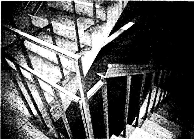
Fig. 8. Typical exterior handrail showing section of extruded stainless steel grip rail. A neat condensation of Kahn's concern for the fluent balancing of function and fabrication.
