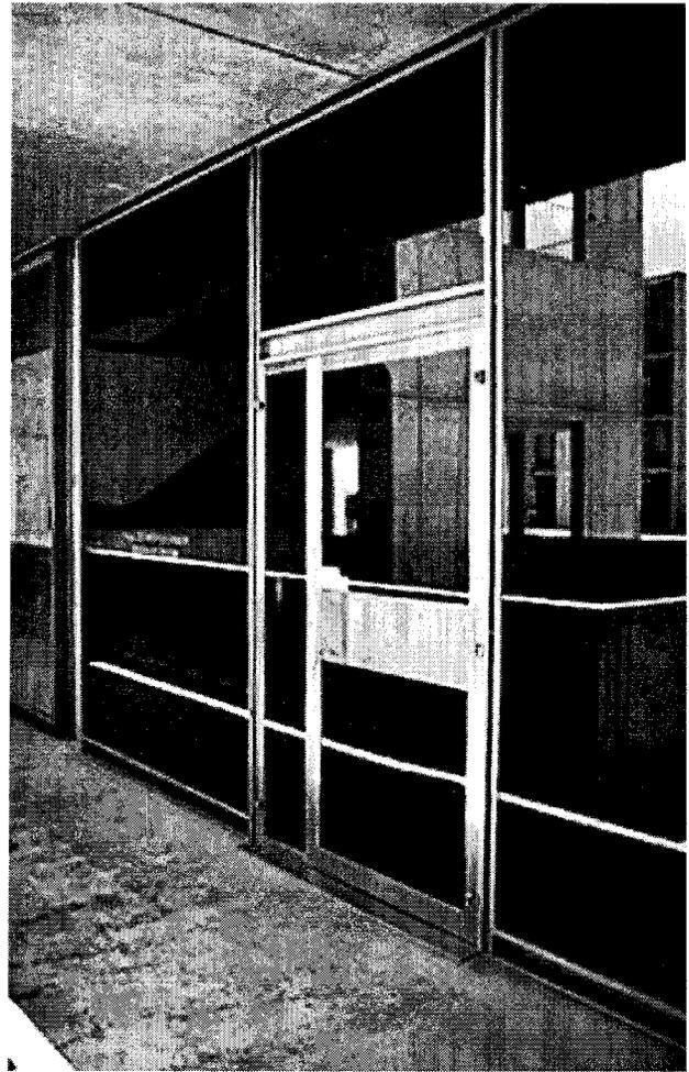
*Fig. 7. Laboratory curtain wall, typical module. Brake-shaped stainless steel forms all major structural elements, supporting large sheets of plate glass. Each door could be changed out through a simple unbolting process from the transom above, or the entire curtain wall module could be removed by unbolting it from the structural columns.*
