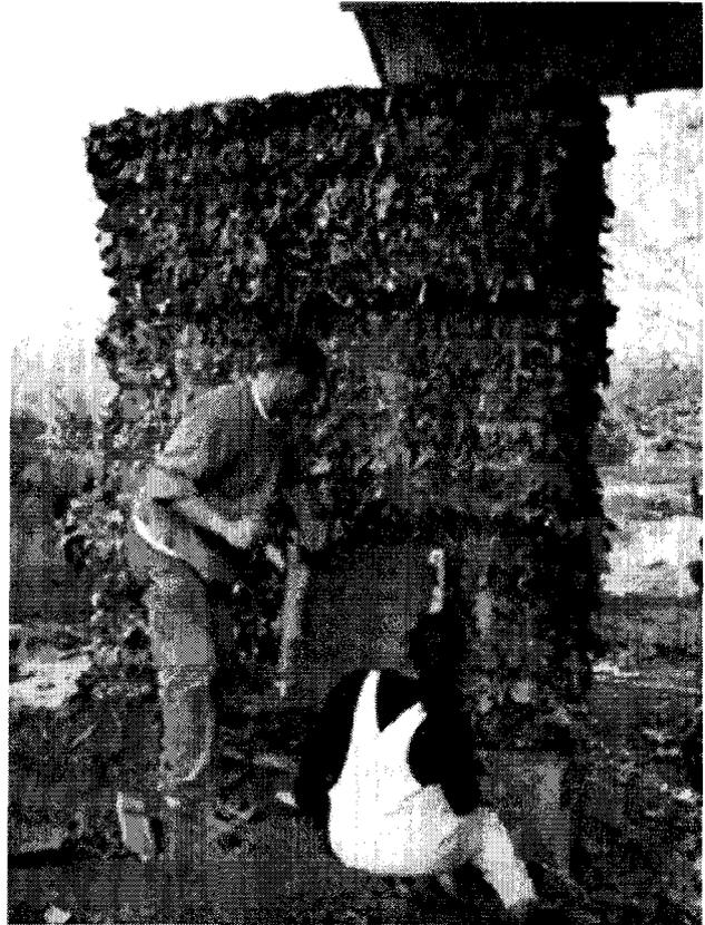
*Fig. 7: Exploring finishing techniques for the corrugated bales*
