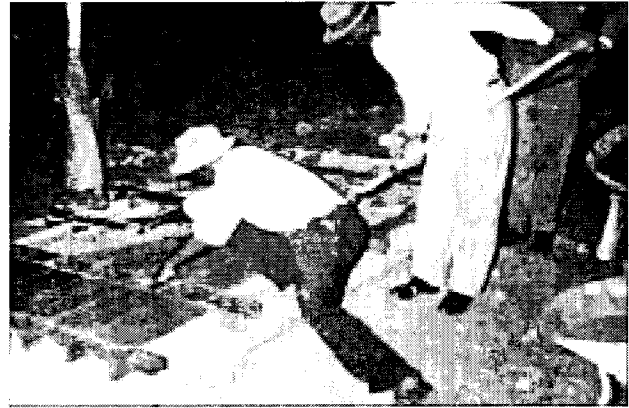
Fig. 8. Using a Wooden Float to Level the Cast Cement. (Source: Low Cash-Cost Housing)
