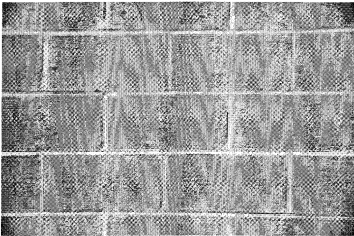
Fig. 16. Standard Concrete Block Wall. (Photo: Don Armstrong)
