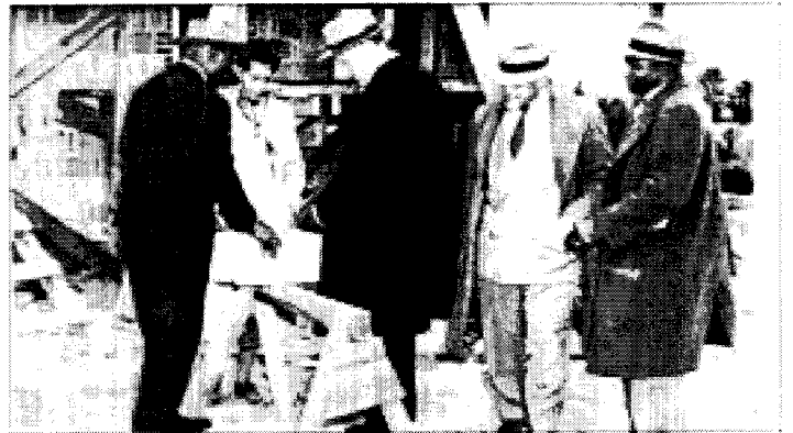
Fig. 4. U. S. Secretary of Agriculture Charles F. Brannan Observing the Laying of Tuskegee Concrete Block. (Source: Low Cash-Cost Housing)
