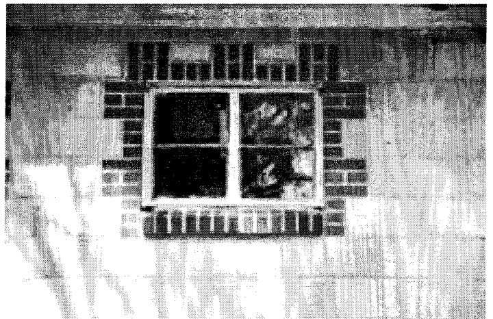
Fig. 18. Tuskegee Block Wall. (Photo: Don Armstrong)
