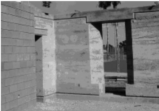
**Figure 19** illustrates the transition from a native technology (rammed earth) to contemporary methods of achieving lateral support (concrete bond beam) and long-lasting structural roof materials (galvanized steel).
