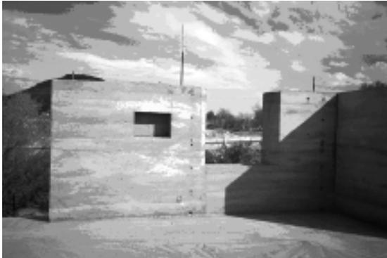
**Figure 18** illustrates the transition from a native technology (rammed earth) to contemporary methods of achieving lateral support (concrete bond beam).
