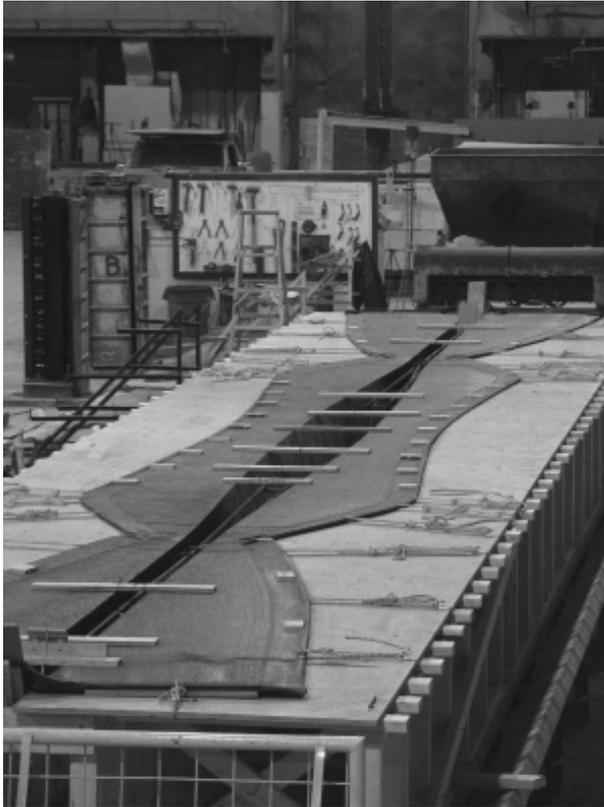
Figure 3. Installation of fabric formwork sheet.
