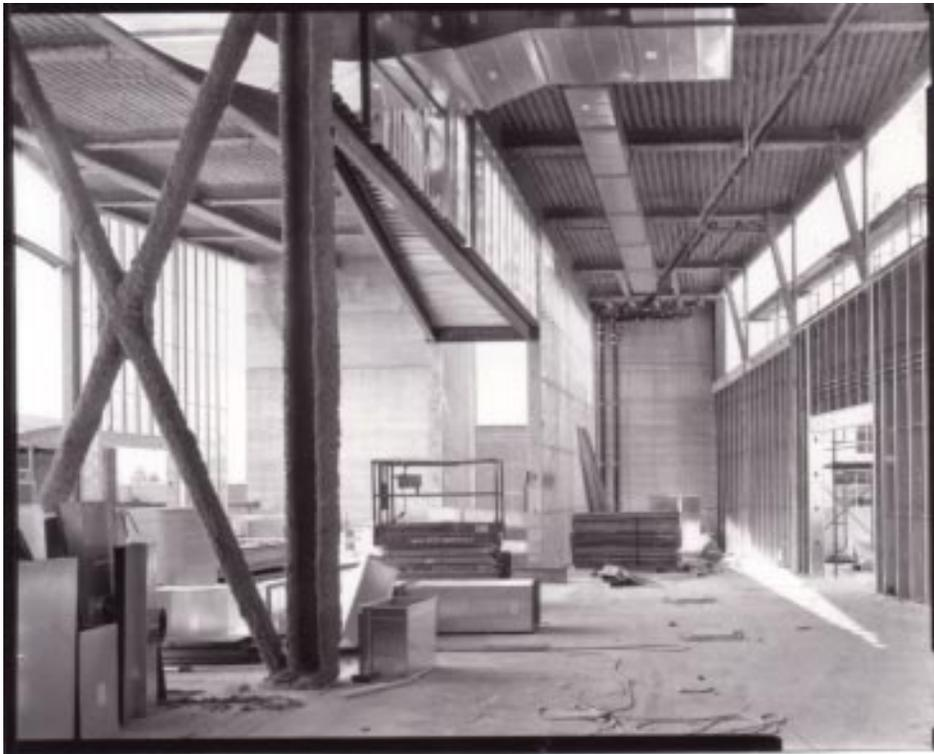
*Figure 5. Milwaukee Art Museum, Milwaukee, WI. Construction of A-frame structure which will later support the building's signature wings. (2000-8.3-9a).*
