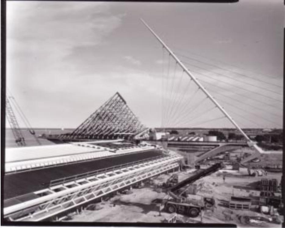
*Figure 6. IIT McCormick-Tribune Campus Center, Chicago, IL. View looking north in main corridor before roof framing is installed. (2002-8.10-22a).*
