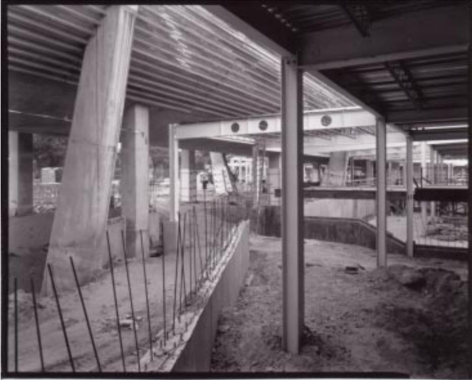
*Figure 7. IIT State Street Village, Chicago, IL. Concrete structure of southern unit reaches its final height. temporary wooden posts, visible on all floors, support the concrete floors until they reach their final hardened strength. (2002-11.3-22a).*
