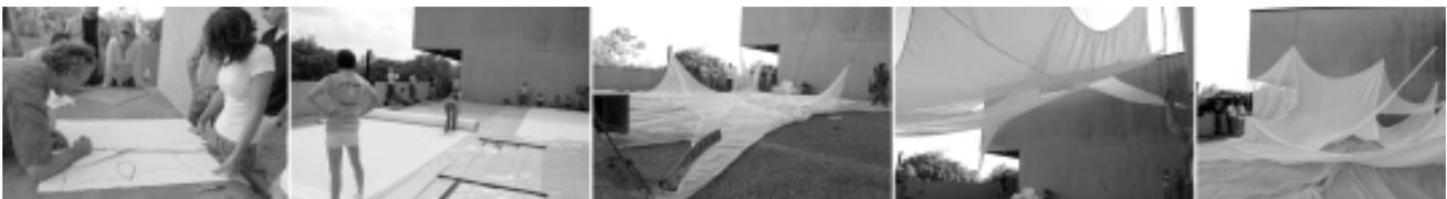
Like the steel, the fabric's form evolved from its bias. The weave of the fabric exerts an equal pull when organized along its diagonal— a condition literally called its bias. As lines of force are identified at the edges, the field begins to move from a loose description (lufts and ripples) to a precisely described complex form (taut). The surface disturbance in the fabric registers its closeness to its ideal form, given its edge condition. The fabric provides feedback.
