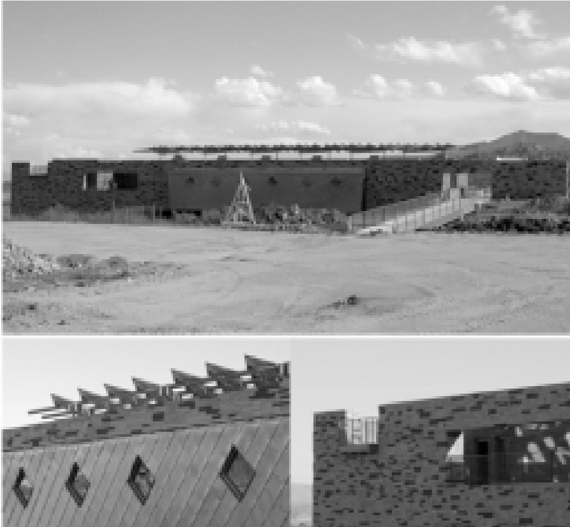
facing wall. Here, in April 2004, the panel tilt angle is still not fine-tuned to its winter position. Even with the panels not exactly in their final position, it is evident that the structure is creating some very characteristic patterns of light and shade on the walls of the main circulation space and patio. The changing configurations of lit and shaded figures are visible through a large opening in the north-facing wall, where one looks into the public patio.
