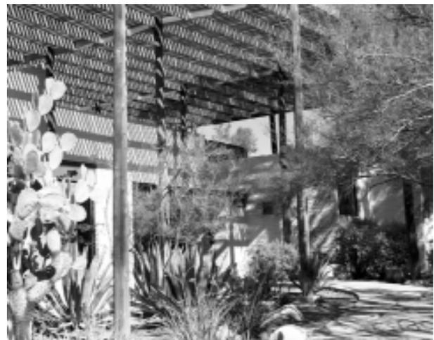
In his Ventana Vista School design, also in Tucson, Arizona, Antoine Predock creates outdoor patios and walkways protected by shading structures assembled from additive sheet metal units. Here the shading devices are conceived of as separate entities that occupy spaces between building volumes while still holding design features integrated with the overall design, see Figure 5.
