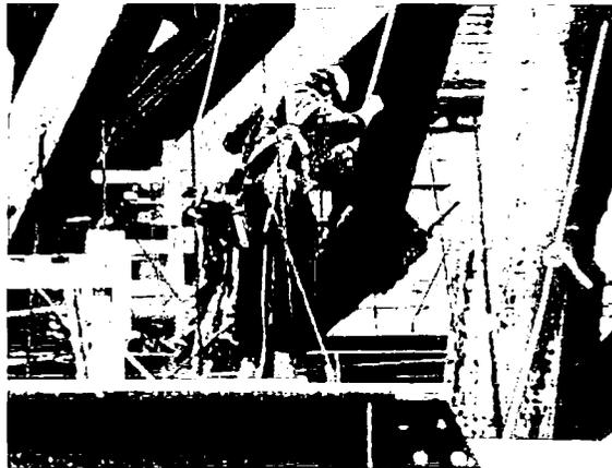
Figure 7. Ironworkers attempt to connect a sloped assemblage of the diagrid
