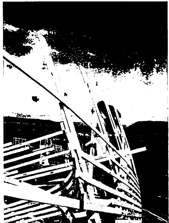
Like a boat swinging downwind of its anchor, prow into the wind, the theatre is anchored at one entrance by a playground slide. It's a permanent theatre, "transparent to the wind," heavy enough to be anchored on the site, yet perforated to reduce the extreme wind load. The theatre has rocks in its pockets: river
