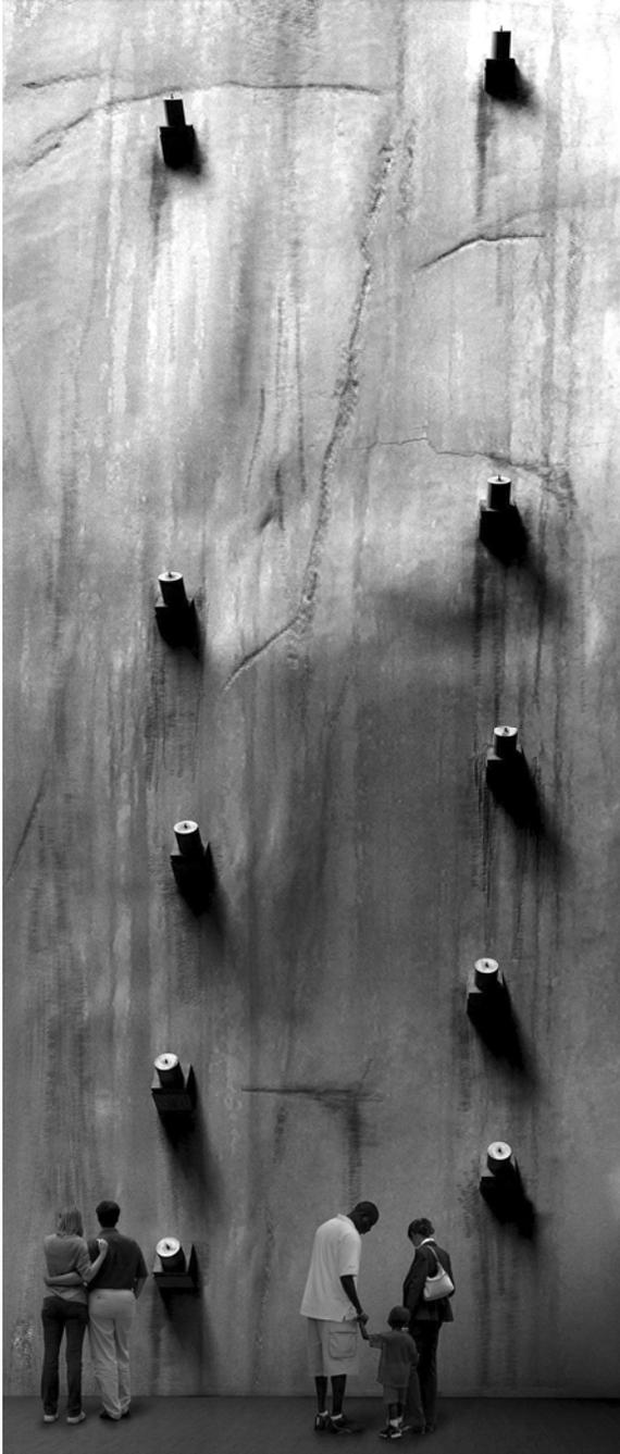
Fig. 4. Rendering of the WTC slurry wall
