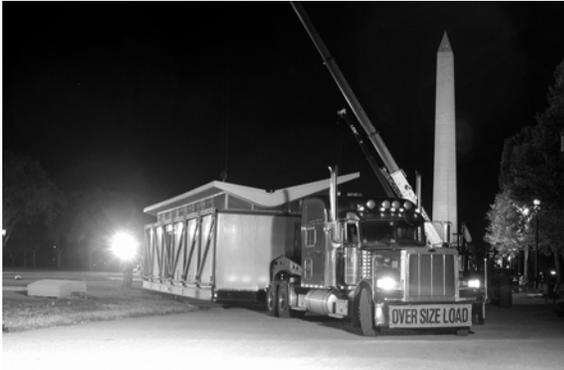
Fig. 2. The house arrived on the mall at 2 a.m. By noon, the house was fully operational. Trusses in the vertical position for transport eventually fold down to become the framework for a cedar wrap-around deck
