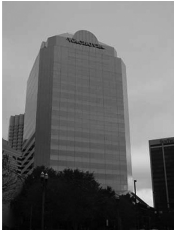
Fig. 1. Enterprise Center, Jacksonville, FL – a typical contemporary building with a typical enclosure system.
