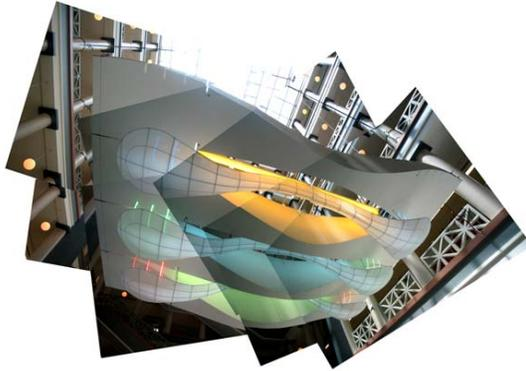
components of this system were derivative of the fabrication tactics and local resources uncovered in the first half of that semester. Primary elements – beams – were conceived as sculpted solid forms, complex shapes that are simple catenary expressions of a uniform load over a simple span. These beams, 15 feet long and 30 inches wide, are sculpted in 2 axes by a CNC controlled hotwire which is typically used to make architectural cornice shapes.
