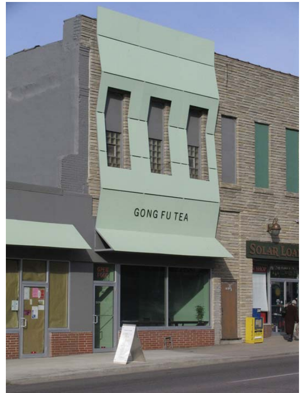
Fig. 2: Multiple layers of façade over brick. Des Moines, Iowa
