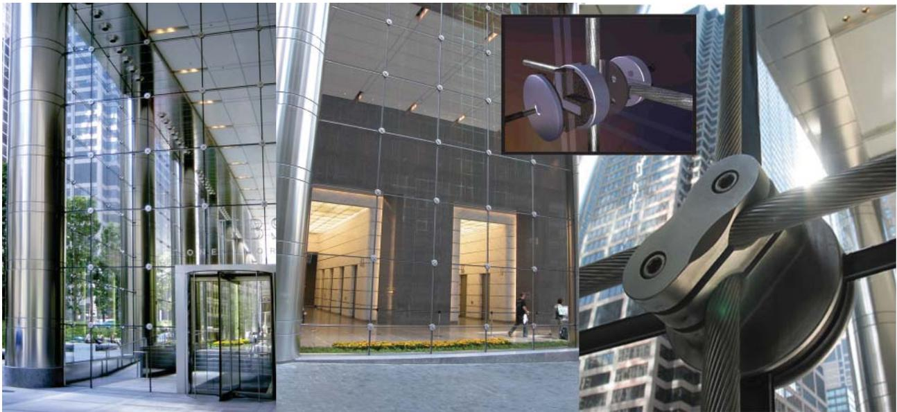
Fig.4: Cable nets top the transparency chart. Here a four-part cast stainless component clamps the cables of this flat 2-way flat cable net and clamps the glass to the net.<sup>6</sup>
