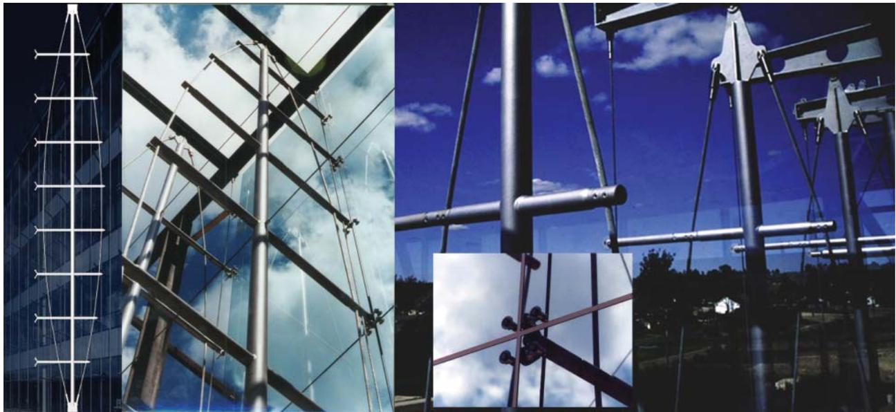
Fig.2: Monolithic glass panes are being attached to the spreaders of these mast trusses. A vertical dead-load cable supports the spreader struts just behind the glazing plane. In this case, horizontal glass will be installed at the top of the trusses back to the building roof.<sup>4</sup>
