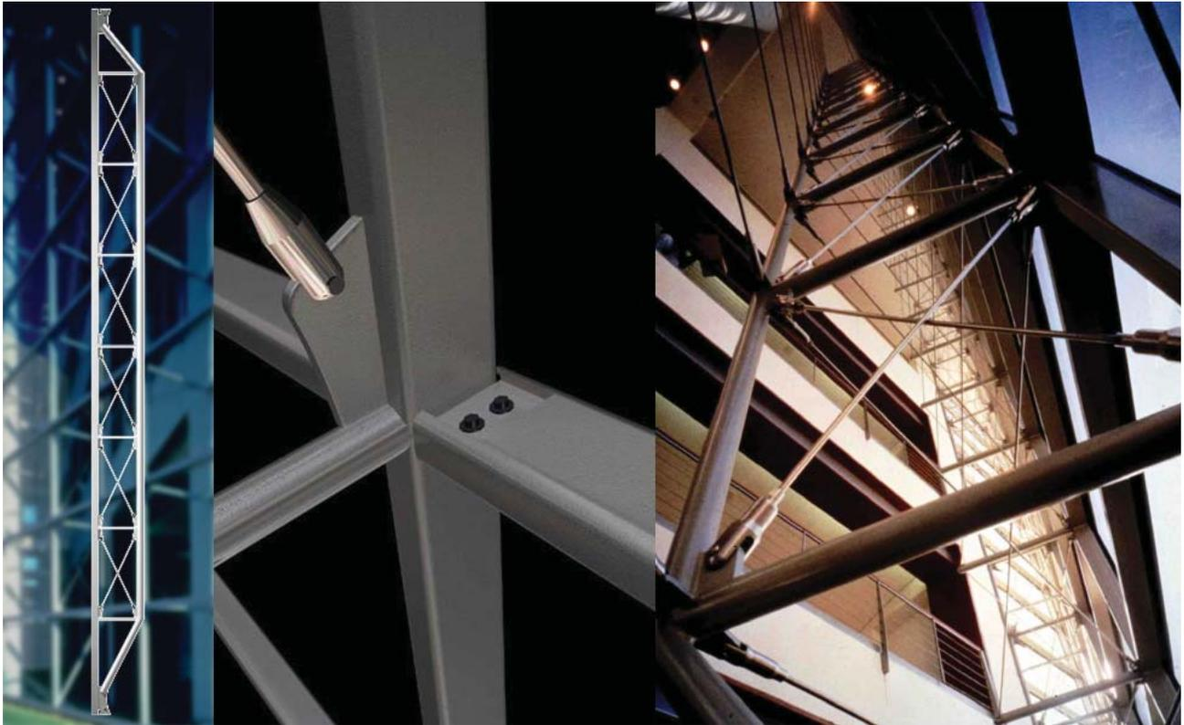
Fig.1: A simple truss system with tension rod bracing and a horizontal purlin mirroring the exterior glazing grid can provide relatively high transparency with considerable economy over more complex truss systems. Virtually any glass system can be adapted to this truss system.<sup>1</sup>
