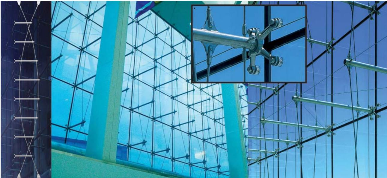
Fig.3: A series of inverted cable trusses define this glass façade. The spreader struts are the only compression elements in the system. Truss stability is achieved by prestressing the cables against the top and bottom boundary supports.<sup>5</sup>
