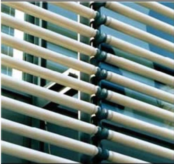
Figure 12 The H2 Glass tubes leave eye-level openings in the barred curtain wall so occupants have unobstructed views. The glass tubes bounce some sunlight onto ceilings bringing light deep into the interior.
