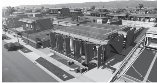
A proposal for an entire neighborhood of mobile houses, each comprised of two similar structures mounted on crane rails. The individual units of each house can be relocated relative to one another or in relation to a striated lawn deck, allowing them to customize their solar exposure or their adjacency to particular exterior conditions at will. (Image: Jones, Partners: Architecture)
