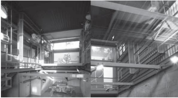
A house with a rolling bridge that can be repositioned within a large open volume. It provides access to the storage shelves on either side, but its guardrails can also fold down to extend its floor area, allowing it to serve as a movable seating area or sleeping loft. (Image: Jones, Partners: Architecture)
