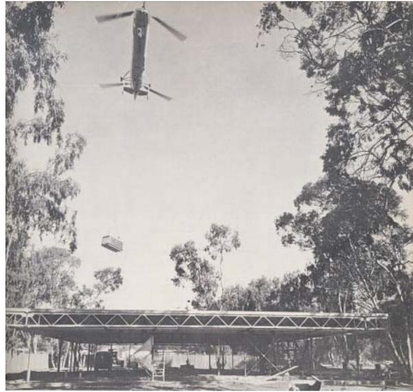
Fig. 4. Prototype construction with aerial component delivery. King, Johnathan "An Industrialized School System for California." *Canadian Architect* 12 (1967): 38.
