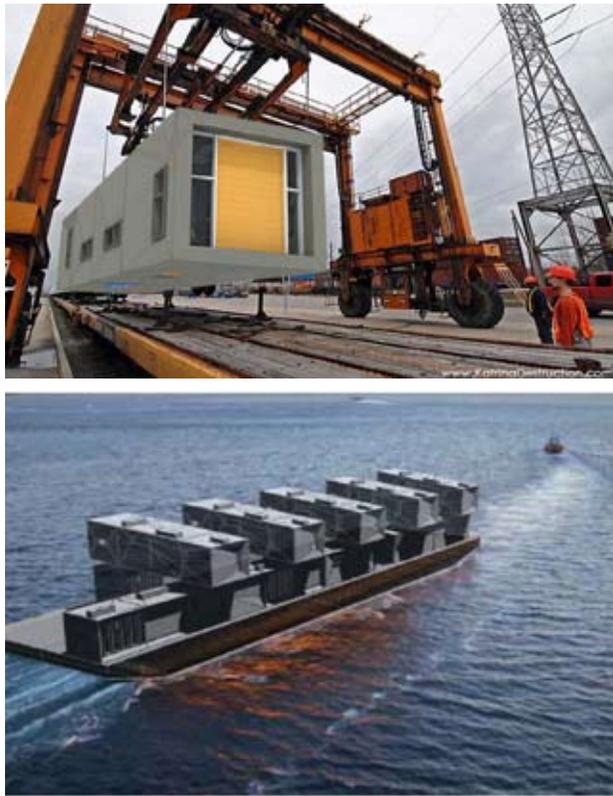
**Figure 3** Gantry cranes install units, barge neighborhood is towed to site
