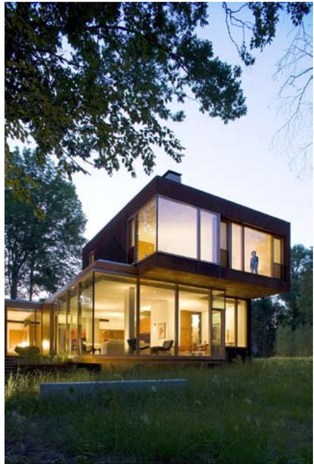
The prismatic volume of the second floor cantilevers over the glass-enclosed living room (above). Floor Plans (left). Section looking north (below).
