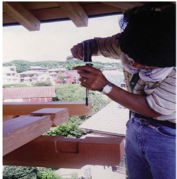
Figure 1. Carpenter cutting joinery
