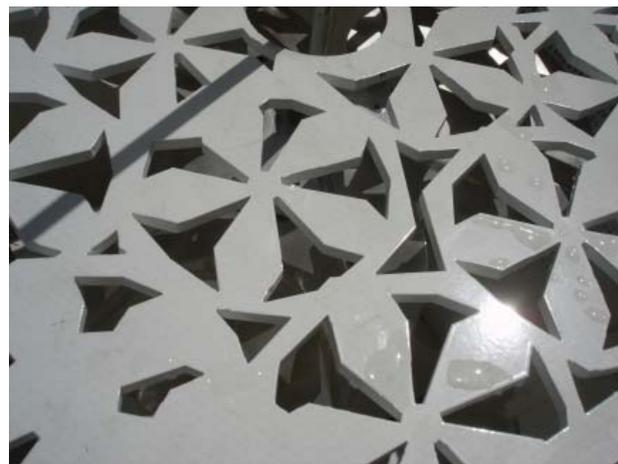
Figure 5. Laser fan pattern functions to allow passage of cooled air through the steel table and to reduce thermal mass.
