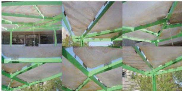
Figure 6. Roof structure and perforated panel pattern from standard steel section
