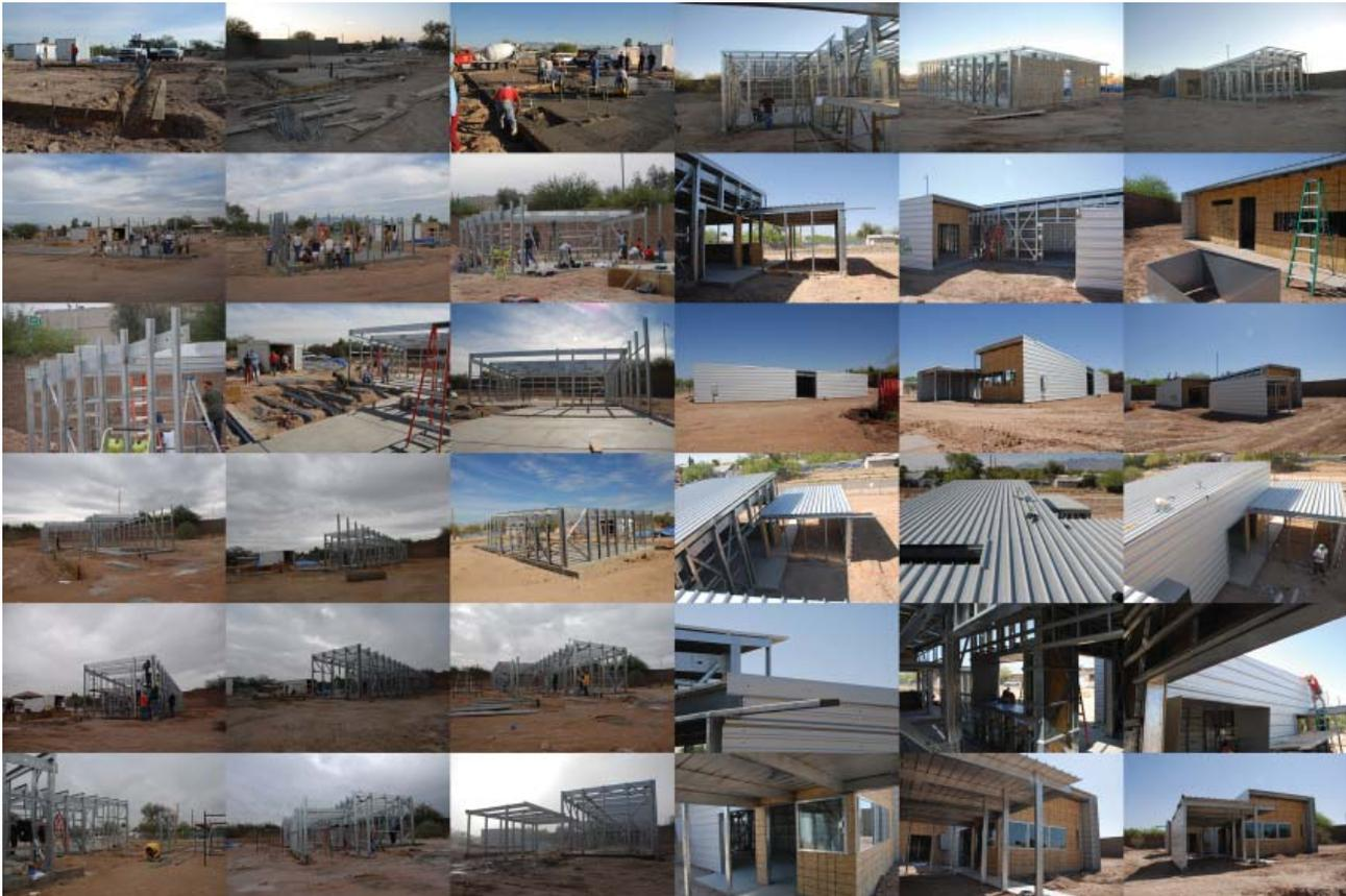
Figure 3. *Civano Demonstration Project*, Construction Sequence for Composite Construction Prototype 3 with students.
