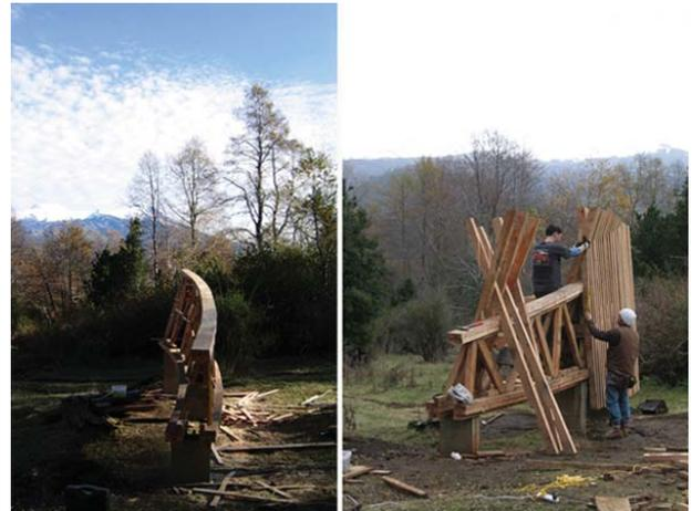
Figure 6. Curved truss + interlocking wall members
