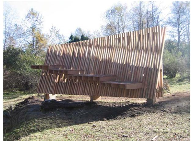
Figure 7. Integrated cantilevered platform supports
