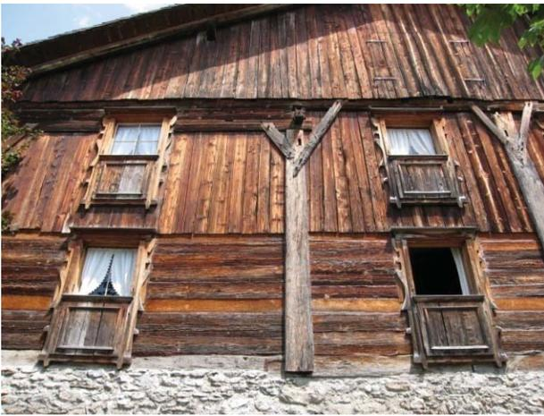
Figure 1. Post-and-beam construction, Sulz
