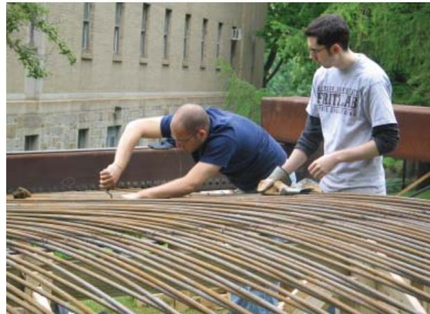
Figure 7. Lehigh students preparing rebar for welding during installation
