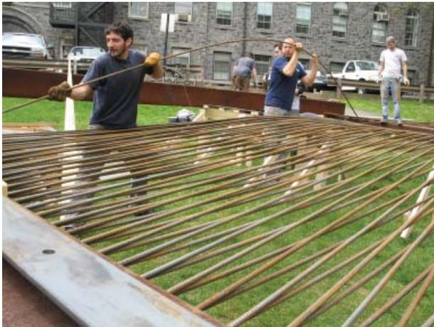
Figure 8. Help from friends and students from Buffalo to thread rebar into the perimeter steel beams
