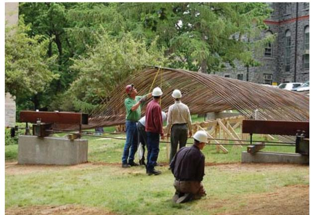
Figure 3. Testing height and deformation during installation of structure on site
