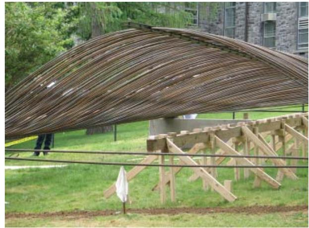
Figure 9. "rebar" takes life as post tensioning rods pull the two perimeter beams together
