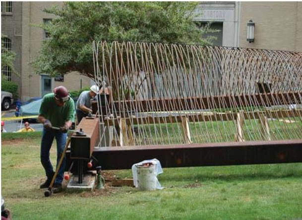
Figure 10. Post-tensioning rods applied to front opening of the grid and slowly cranked.
