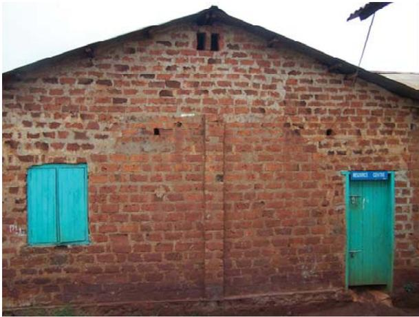
Figure 1. Typical hut built with adobe construction and typical mud-brick construction
