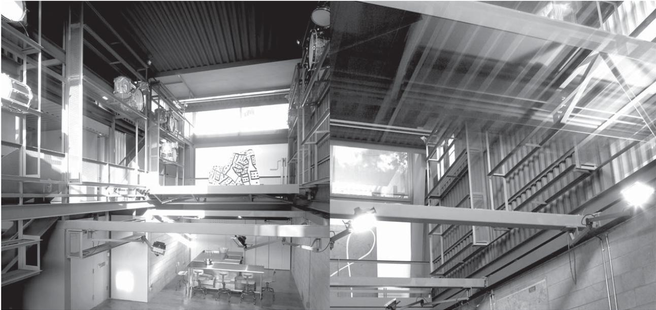
Figure 1. This residence includes a movable mezzanine that can be rolled along the length of its main volume, and can be joined with a small street-facing balcony to make a larger indoor/outdoor space. (Jones, Partners: Architecture)
