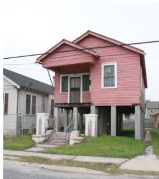
Figure 3. This picture shows both how the neighborhood is changing due to the flood. Houses are being lifted up to eight feet off the ground. This scheme suggests that the resulting space can be used for community activity. This image also shows the shutters closed in anticipation of a storm.
