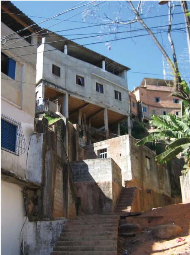
Figure 3. The concrete structure of a regular favela building.
