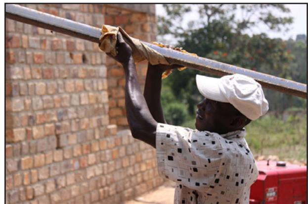
Figure 3: Lifting purlin into place
