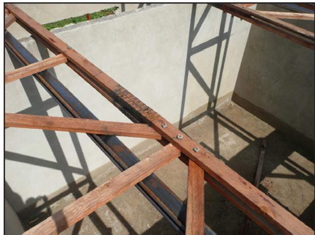
Figure 4: Timber trusses ready for final installation
