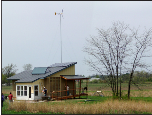
Fig. 4: The Eco Center nearing completion with the alternative energy systems installed
