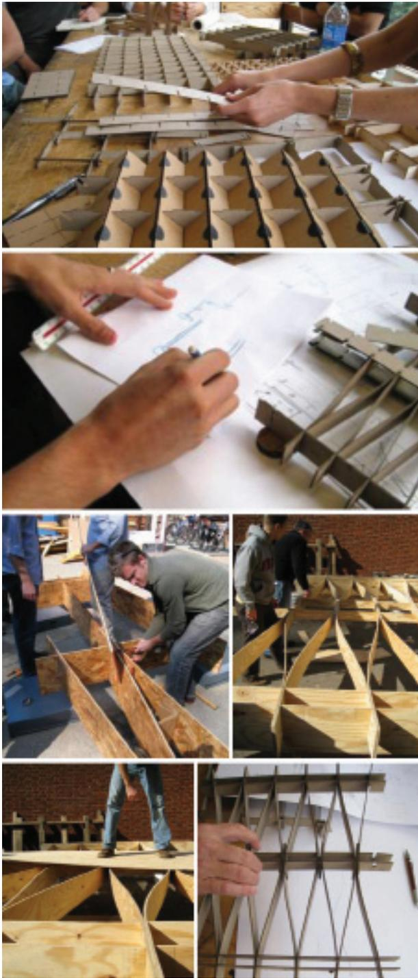
Figure 6: TDRH structural frame fabrication
