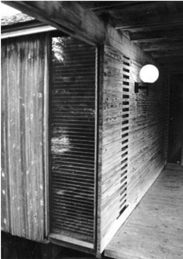
Image 4 – Ventilation strips at wall
