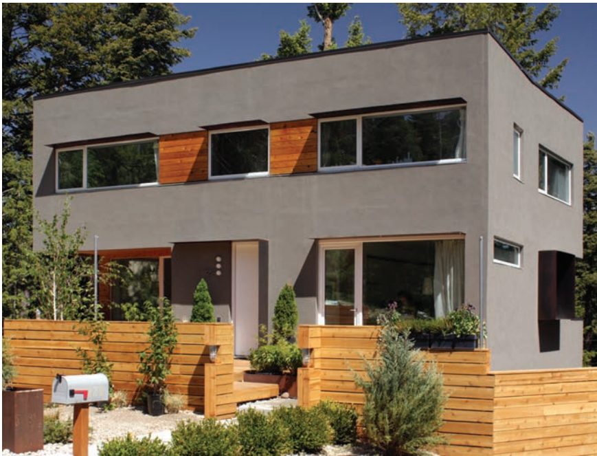
South East Entrance Elevation
