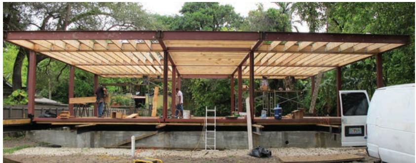
Construction Photo (Miami, FL 2012) - Showing Steel Superstructure
