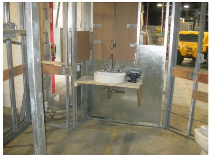
Figure 4. Bathroom pod mockup for the MVH South project (Photo taken by author)
