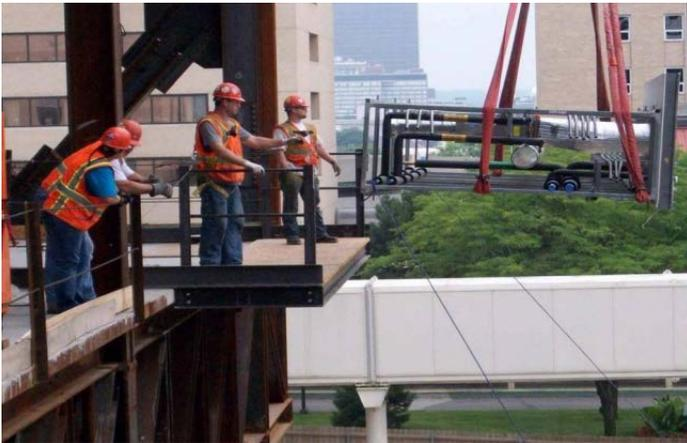
Figure 5. MEP ceiling rack being hoisted to the landing platform with lifting straps (Source: Skanska USA Building)
