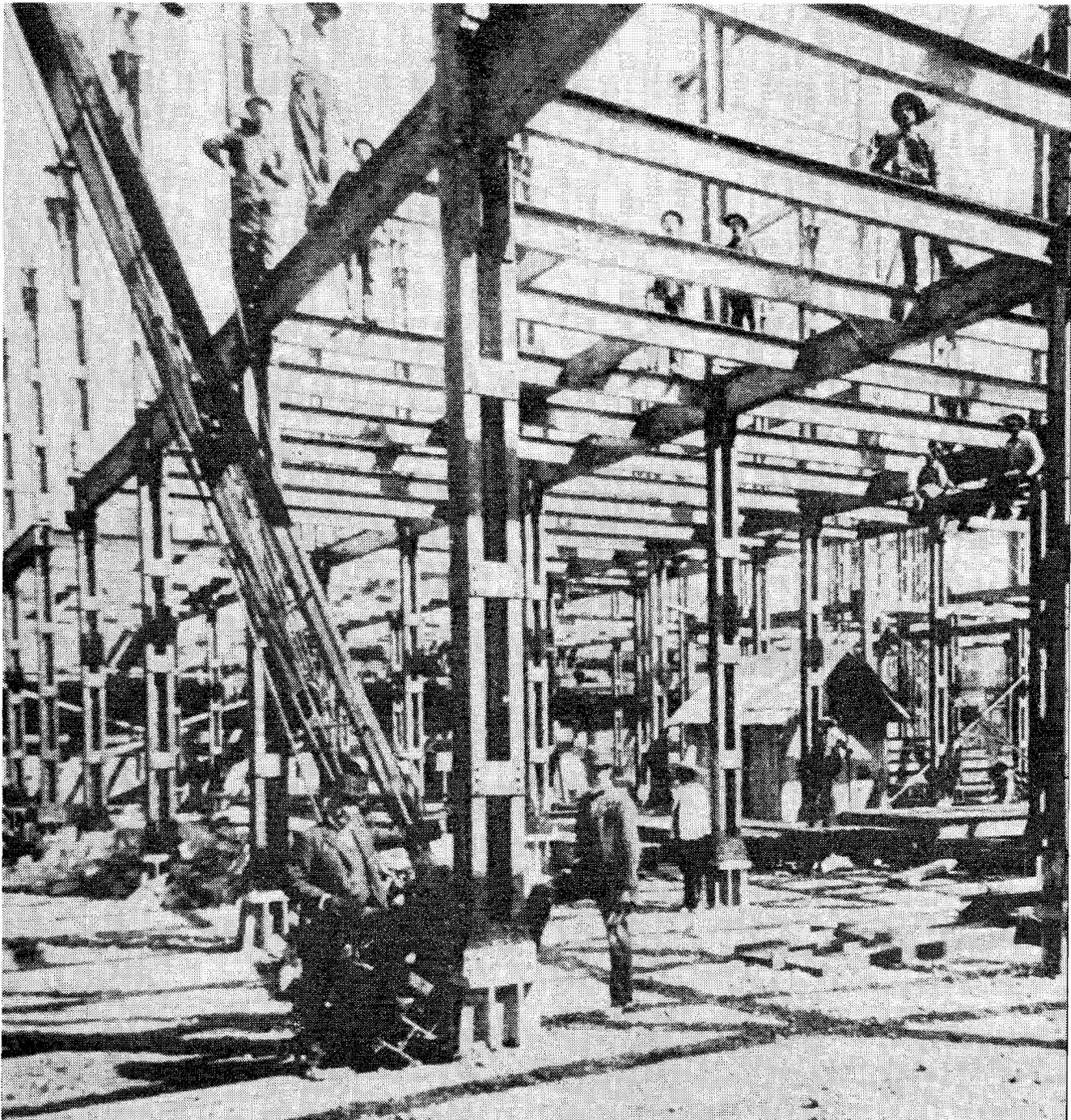
Figure 2. Roberto Boker Building, Mexico City, constructed with prefabricated steel members by the Milliken Company, 1899.
