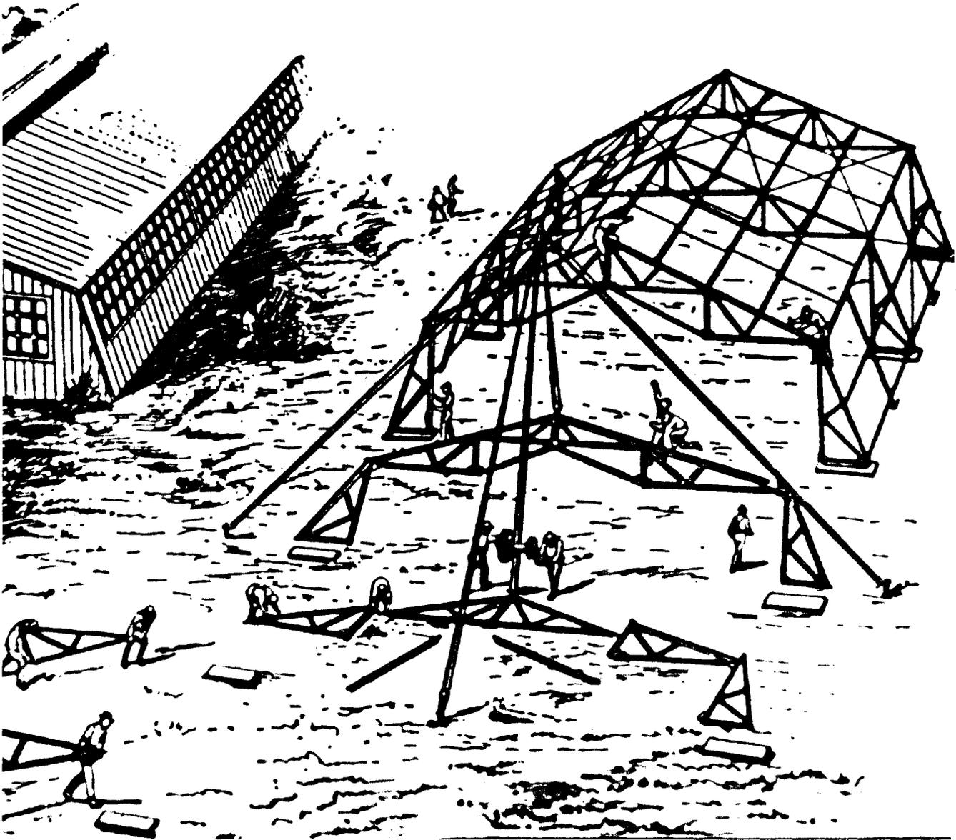
Fig. 3. Erection of a Milliken Building, 1920
