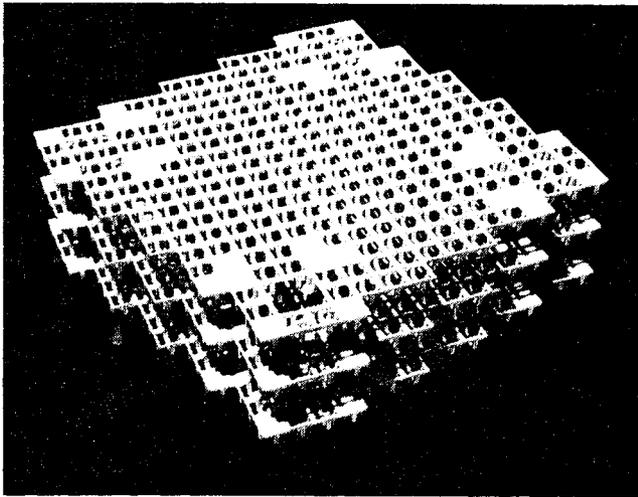
Fig. 3. Coupled Pan Space Frame Construction System: offset grid aligns to both the site and to South.
